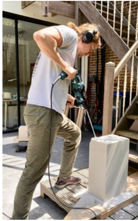
drill the non-planar surface
