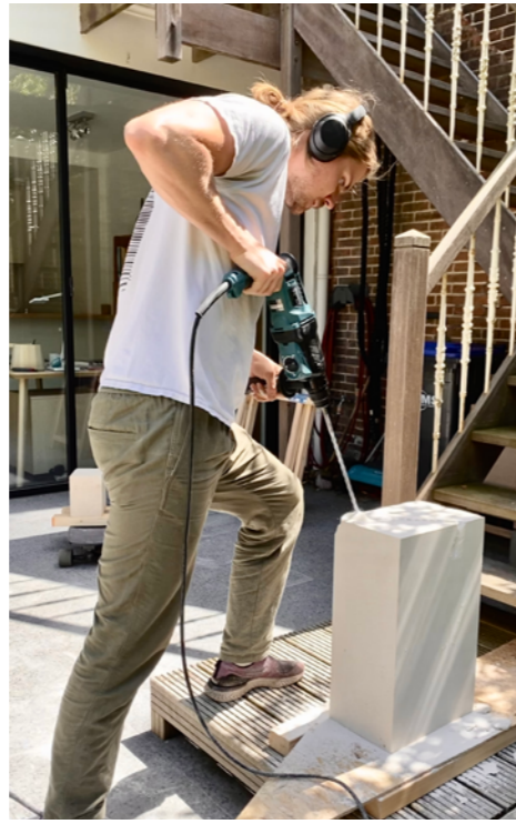
drill the non-planar surface
